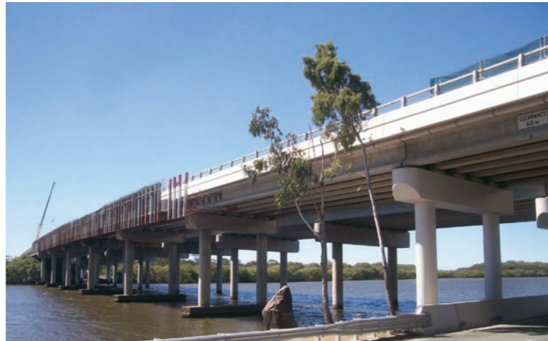
Widening work on the original Maroochy River bridge progresses
