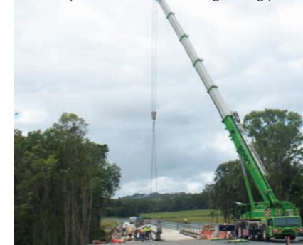
Final span of Eudlo Creek bridge being placed
