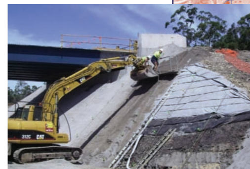
Below: Slope protection works to southern service road bridge abutment
