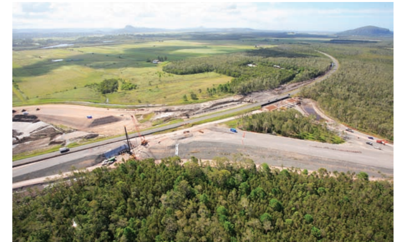
Constructing the new northern bypass at Pacific Paradise
