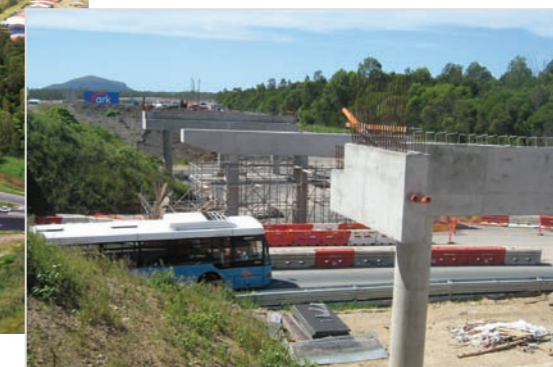
Left: Completed bridge piers at the David Low Way interchange
